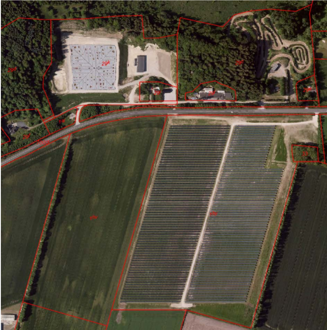
Figure 2: Aerial view on the solar district heating system of Dronninglund Fjernvarme (Source: Brønderslev Municipality). A flat plate collector field (1by) with a gross collector area of 40,466 m 2 hydraulically connected to a 62,000 m 3 pit thermal energy storage (29k) as well as to an absorption heat pump with 2.6 MW th heating capacity for improved operation flexibility was put into operation in 2014. From 06/2015-05/2016 48 % of the annual DH output originated from solar thermal.
