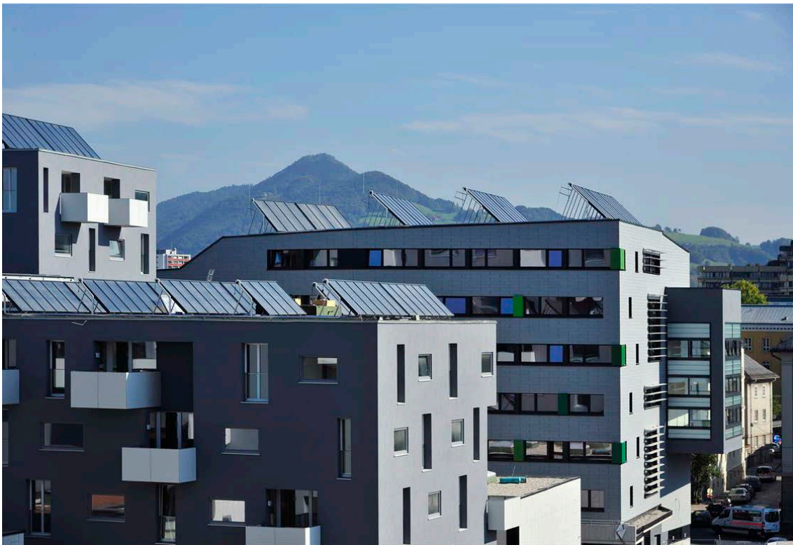
Figure 9: Aerial view on Northern part of the urban quarter “Stadtwerk Lehen” (Source: top: AEE INTEC, bottom: Fotohof). In sum, 2,048 m 2 solar thermal collectors are split into 13 roof-mounted collector fields and roughly supply 25% of the final thermal energy demand (incl. network heat losses) of the buildings with a heated floor area of 48,860 m 2 .
