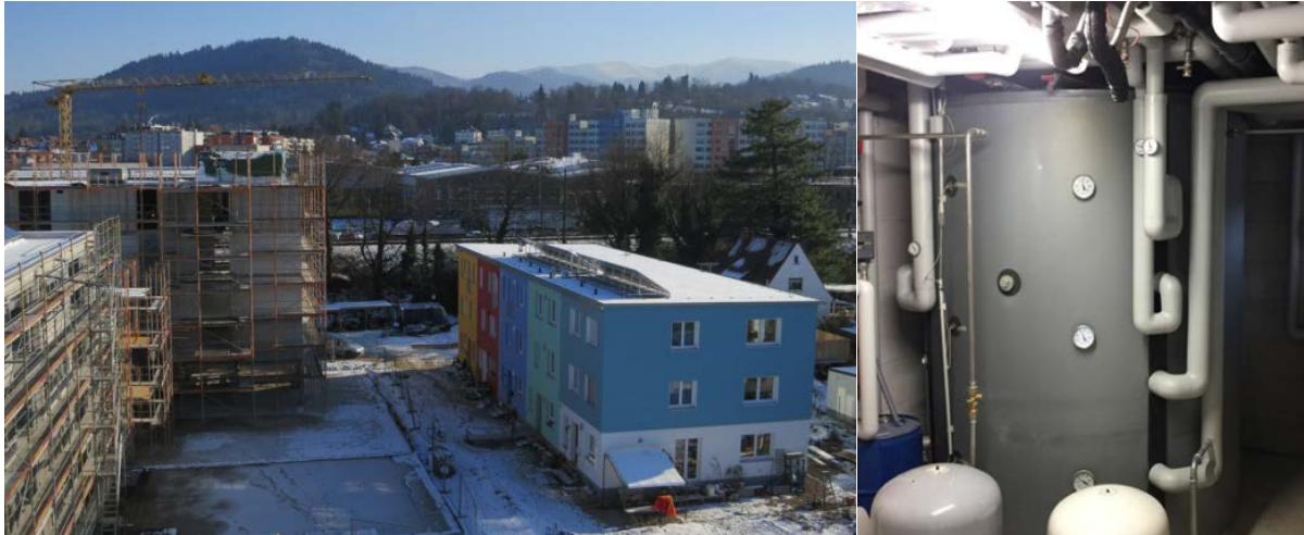
Figure 14: View on Eastern part of the urban quarter “Gutleutmatten” (Source: Fraunhofer ISE). In sum, 2,220 m 2 solar thermal collectors are split into 38 roof-mounted collector fields. The solar thermal system is designed to supply around 24% of the final thermal energy demand (incl. network heat losses) of the new buildings with a heated floor area of approx. 40,000 m 2 .
